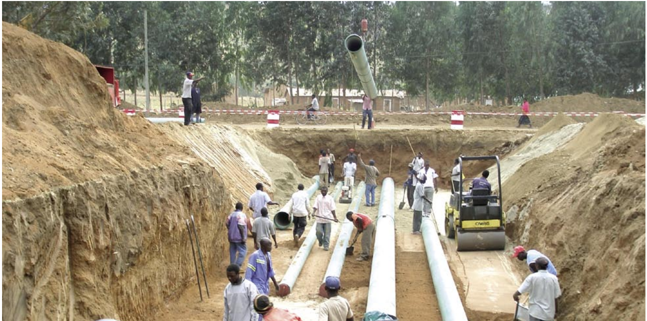
Laying of DN 200 up to DN 500 trunk mains in Iringa, Tanzania
