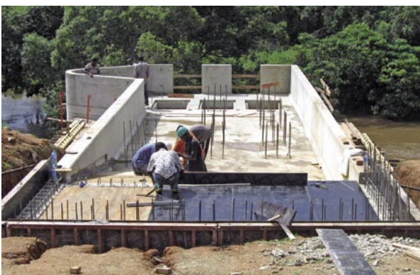
Construction of raw water intake station at Ruaha River, Tanzania
