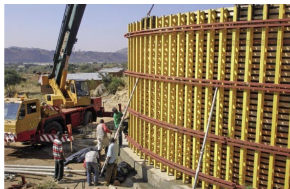
Setting of formwork for a tank wall in Iringa
