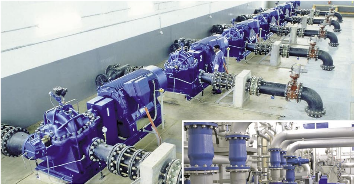
Six pumping sets, each with a capacity of 833 m 3 /h in Kampala, Uganda
