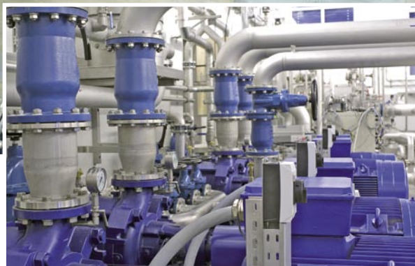
Six pumping sets, each with a capacity of 833 m 3 /h in Kampala, Uganda
